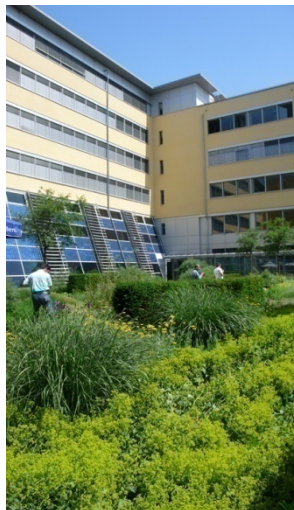
Figure 3. Intensive green roof, Friburg (Germany)
