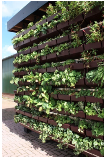
Figure 9. Living wall system based on planter boxes in Benthuizen (The Netherlands), Green Wave, 2010
