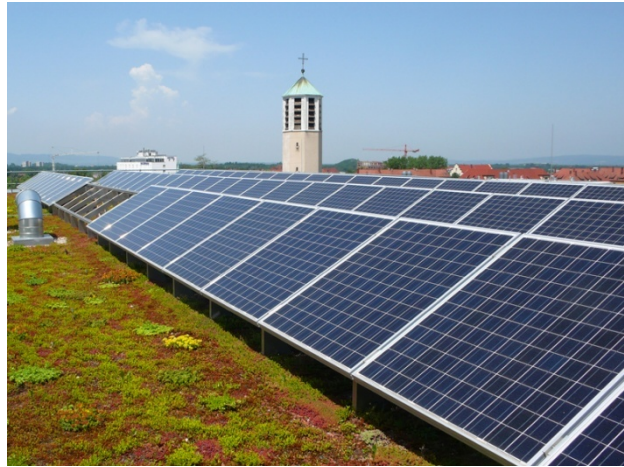
Figure 5. Extensive green roof, Friburg (Germany)
