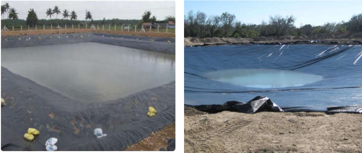
Fig. 16. Lining of farm pond with plastic film
