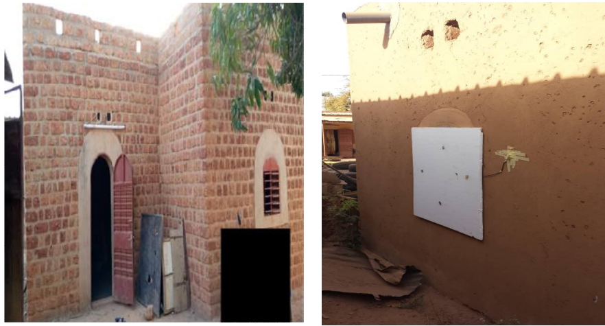
Fig. 1. Image of the East and West facades of the studied building
