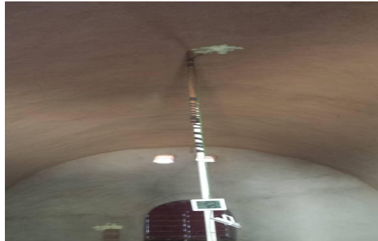
Fig. 3. The vault of the living room seen from the inside
