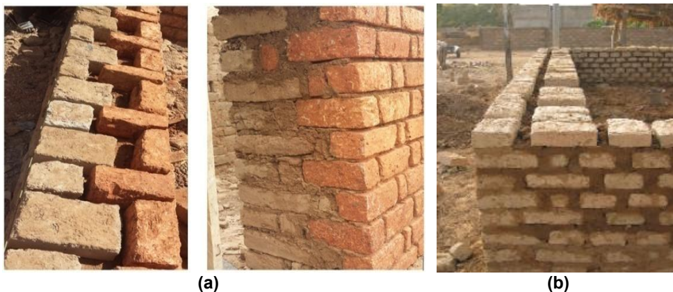
Fig. 4. (a) Image illustrating the mixed structure of the walls on the East and South sides ; (b) Image illustrating a wall bearing a Nubian vault made of adobe [9]
